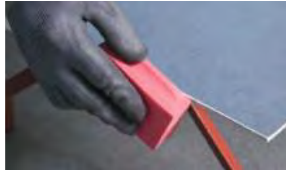
With a diamond sandpaper buffer in diagonal position from bottom to top and never laterally.
